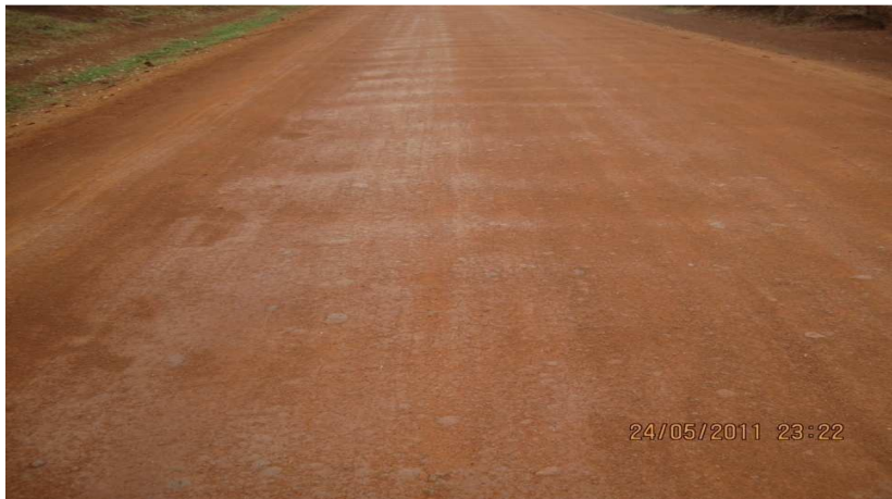
Figure5.1. 1: Corrugated, rutting and crack surface of the road
